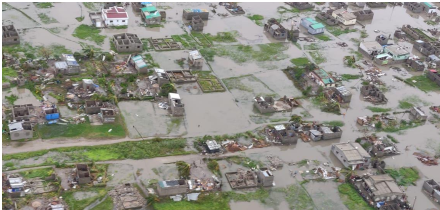
Figure 5.2 Destruction in Beira following cyclone Idai.
